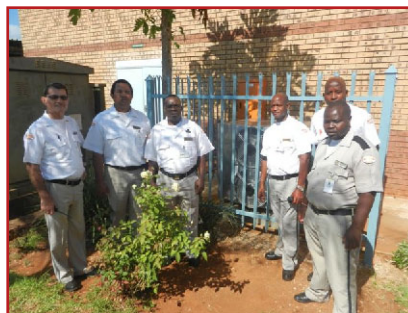
Project team at newly installed heat pump. Left to Right: Johan Wagenaar, Clement Raphalalani, David Makhubele, Lazarus Ncongwane, Azwi Netshiomvani, and Livhuani Mafunzwaini
