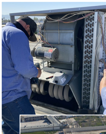
Bi-Polar Ionization units being installed at the Mesa Verde Processing Center
